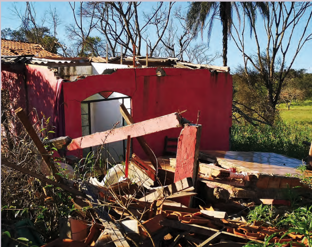
House destroyed by the tailings (Brumadinho, June 2019). © Lavite & Müller-Hoff
